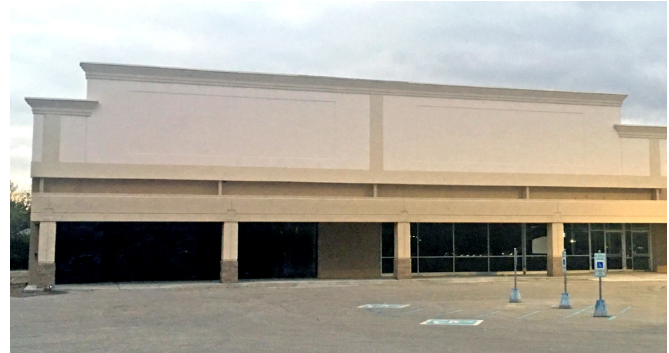
Newly renovated façade
