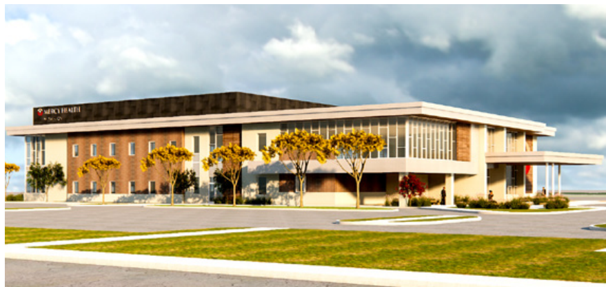
Now Under Construction
