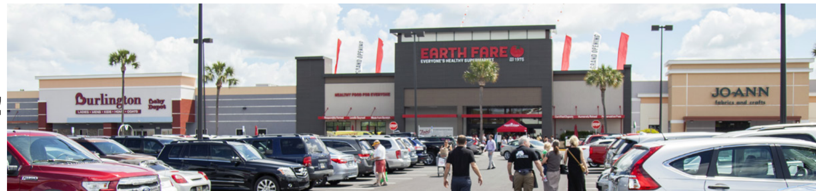
Newly Renovated Facade!
