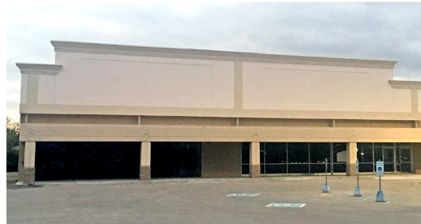
Newly renovated façade
