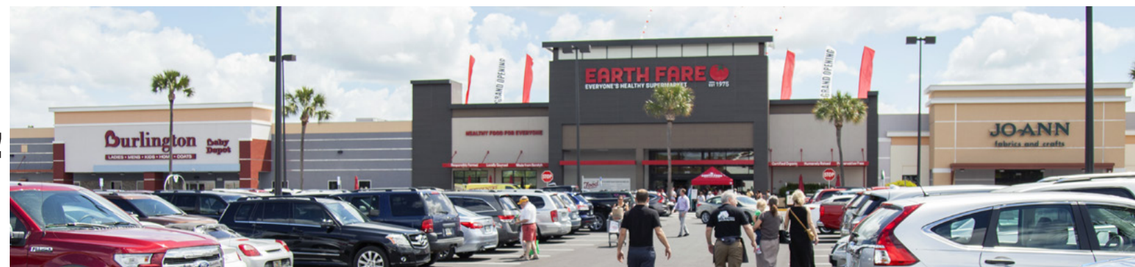
Newly Renovated Facade!
